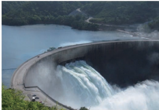
Fig. 6. Downstream view of the Kariba Dam during spillage through three non-adjacent gates in April 2010 (courtesy of B. Goguel).
