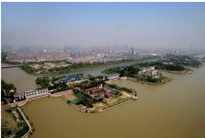
Fig. 2. Jiangu Pumping Station in the East Route Project (ERP).
