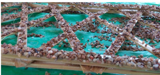
Fig. 2. Lime water treated bamboo mat coated with epoxy and sand.
