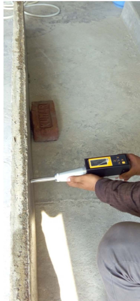
Fig. 4. Rebound hammer test.
