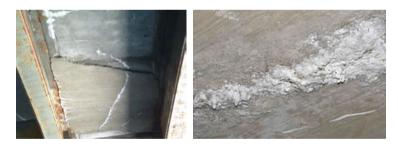
Fig. 6. Leached salts and minerals on concrete surface.
