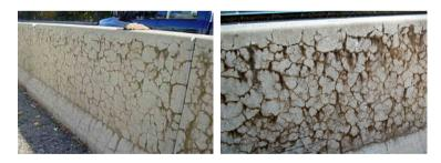
Fig. 3. Degradation by the aggregate expansion paving the way to the further concrete degradation.
