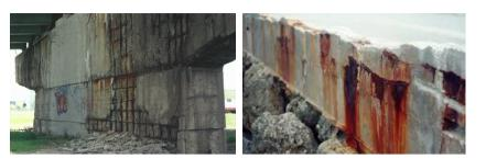
Fig. 8. Reinforcement corrosion of the structure parts in contact with soil.
