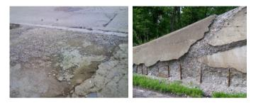
Fig. 4. Concrete degradation caused by crystallization of road defrosting salt.
