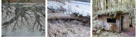
Fig. 2. Degradation of concrete caused by the tree roots and vegetation.
