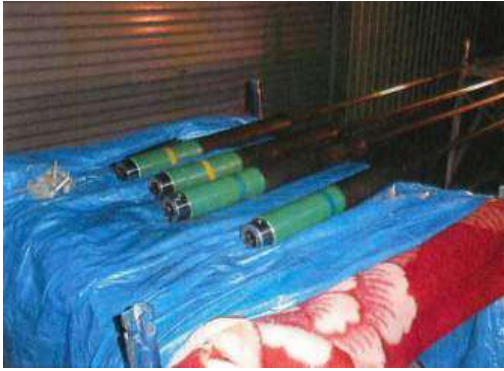
Figure 22. Steel sleeves before Epoxy resin Injection
