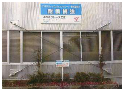
Figure 30. Completion of ACM brace installation
