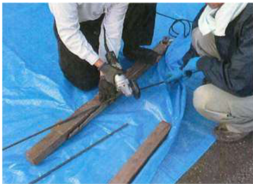
Figure 20. CFRP rod cutting work
