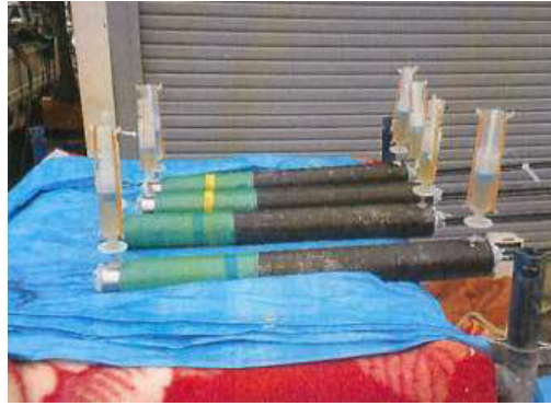
Figure 23. Epoxy resin injection work into steel sleeves
