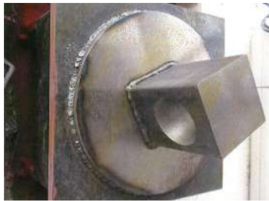
Figure 19. Steel anchor after welding work
