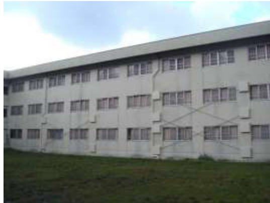
Figure 9. Completion of ACM braces
