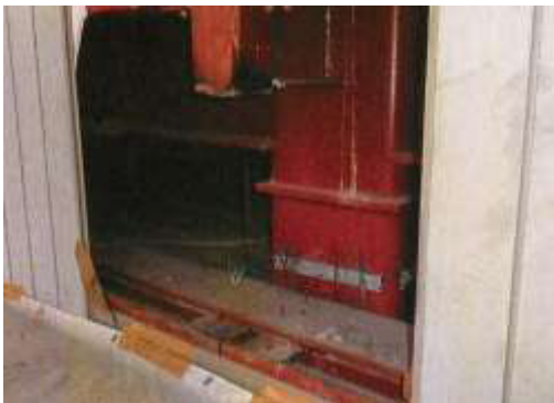
Figure 14. Steel column before ACM brace installation work
