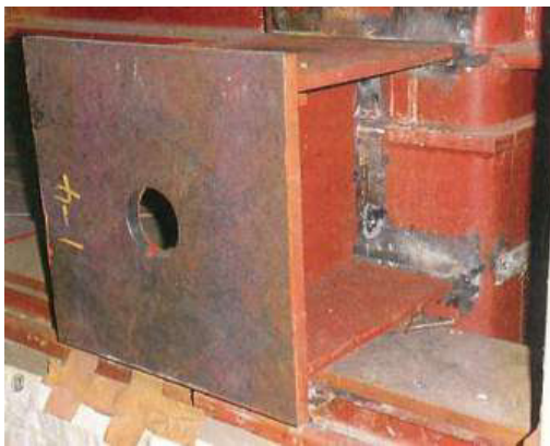
Figure 18. Bracket after welding work
