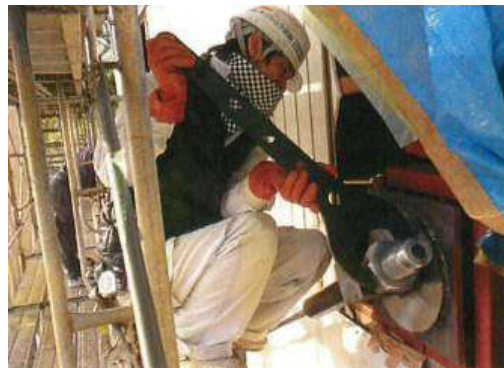
Figure 25. Tightening work of steel-nut with a screwdriver
