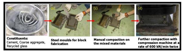
Fig. 2. Glass-concrete paving block making process.
