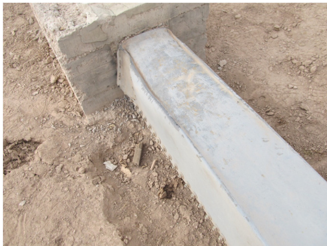
Fig. 15. Plastic strain in steel jacketing.
