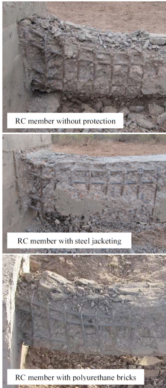
Fig. 14. Detail of the damage suffered by the members for the blast load.
