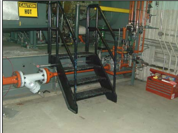
4" Y-strainer (Left) 2 nd Cut Regulator (Right)
