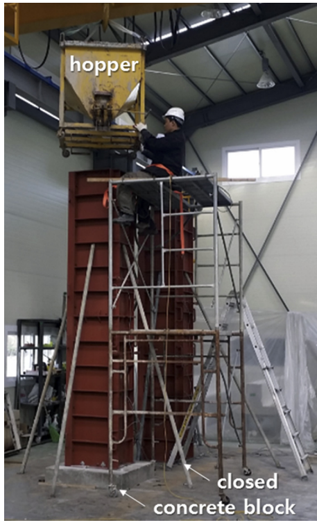
Fig. 2. Picture of placing process of the mockup test samples.
