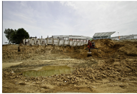
Fig. 4. Photo during the construction of the frames.
