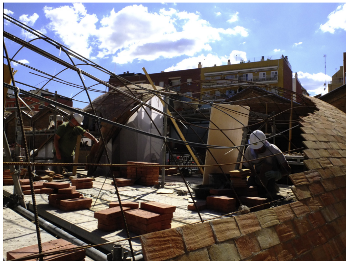
Fig. 7. Grid of bent steel rods. © Manuel de Lózar and Paula López Barba.
