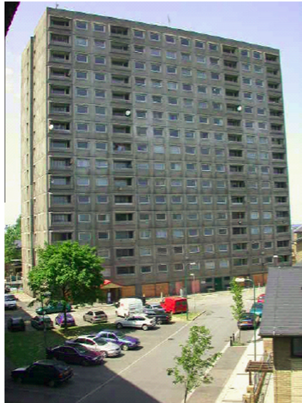
Fig. 5. The Hiscocks House at Stonebridge Park (Tower A).
