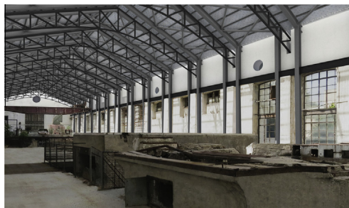
Fig. 4. Render of the new pairs of steel frames aligned symmetrically with the existing steel truss girders in building A.
