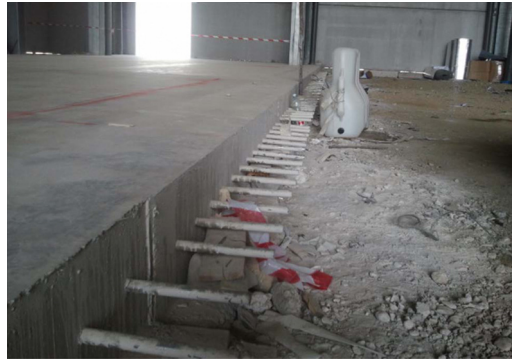
Fig. 11. Photo of the first examined surface without treatment (Floor No. 1).
