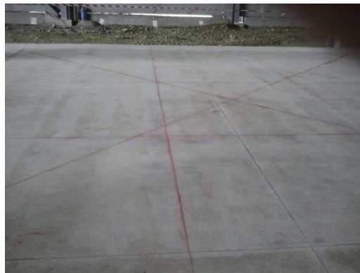
Fig. 12. Photo of treatment by means of surface grinding (Floor No. 2).
