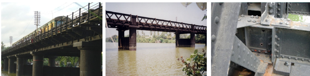
Fig. 1. General views of the riveted railway bridge.
