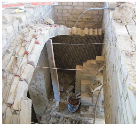
Nubian vault built without formwork
