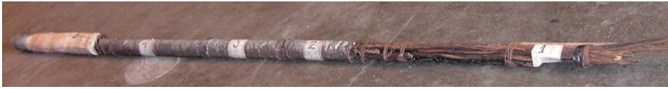
Fig. 1. Damage cable part (subject of this study) matched inside the anchor, with a length of 1950 mm.
