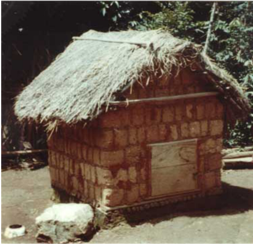
Fig. 4. Used as a roofing element and structural base in mud house (Anon., 2015b).
