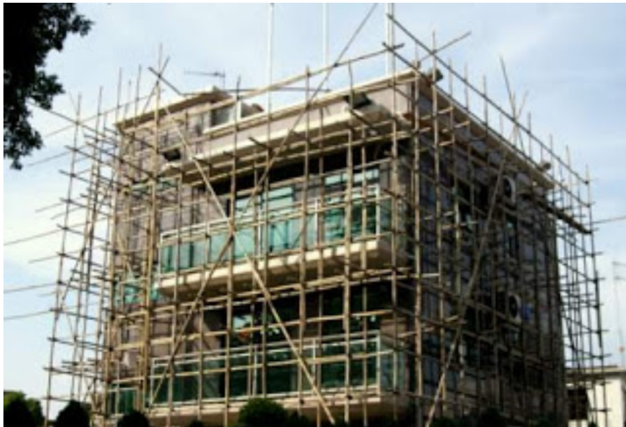
Fig. 5. Bamboo used for scaffolding (Anon., 2015f).
