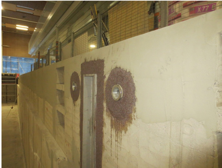
Fig. 6. Epoxy-based materials were used to seal all penetrations.
