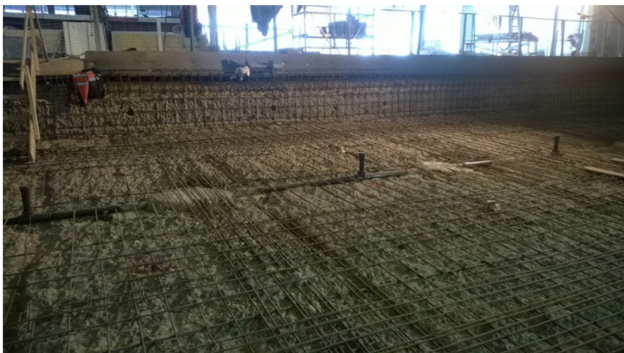
Fig. 5. Upper reinforcement of ground slab. New water treatment pipes were installed before reinforcement.
