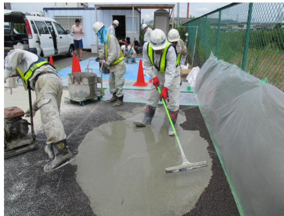
Fig. 4. Construction of the CBGMs.
