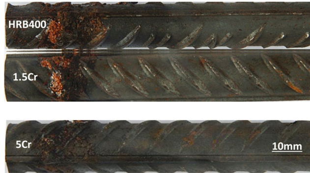
Fig. 7. Corrosion morphology of anodic rebars after a 15-week macrocell corrosion test.
