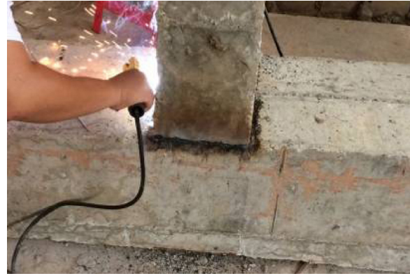
Fig. 1 – Electric welding of a welded plate joint.
