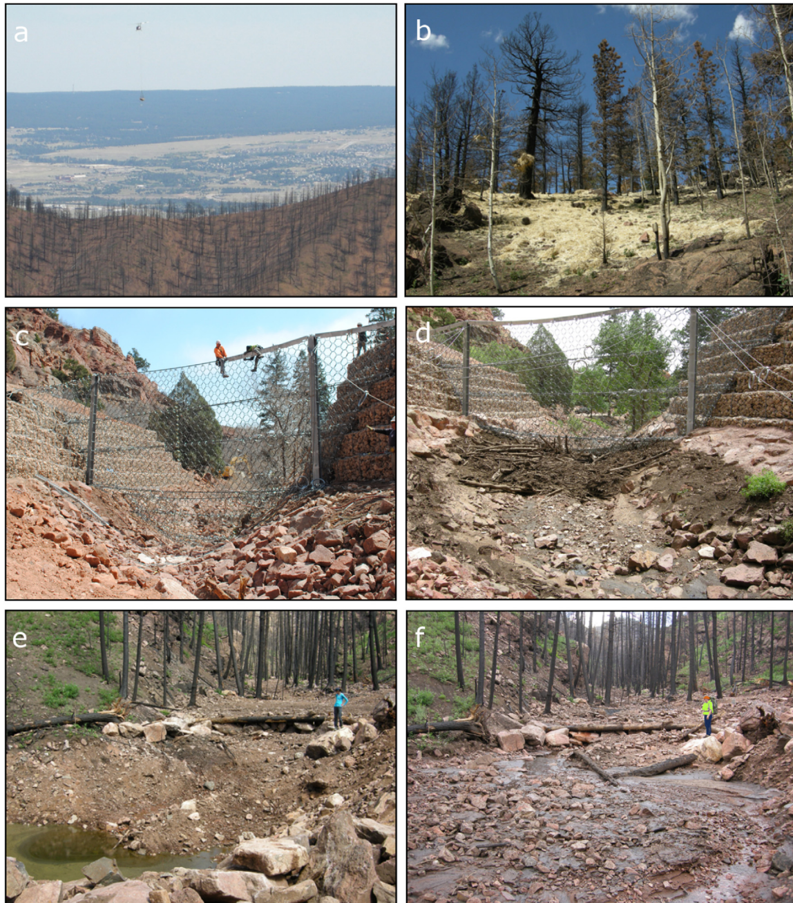
Fig. 4. Human responses to Waldo Canyon Fire: (a) aerial mulching after containment of fire (helicopter is seen in sky, top left of center; photo taken 16 September 2012) (b) straw treatment from aerial application (photo taken 16 September 2012) (c) sediment fence over 6 m (20 ft) tall, constructed upstream of residential community (photo taken March 2013 showing construction workers on fence); (d) sediment and wood behind fence after storm (photo taken 6 July 2013); (e) in-channel modification: sediment basins (photo taken 30 June 2013); (f) sediment basin filled after storms (photo taken 13 July 2013).
