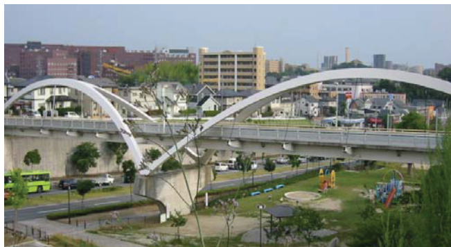
Figure 8. The full view of the Bridge
