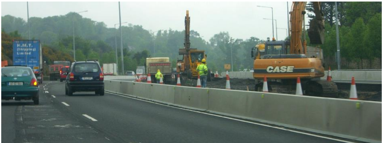
FIGURE 5 Work zone protection at level N2/W4
