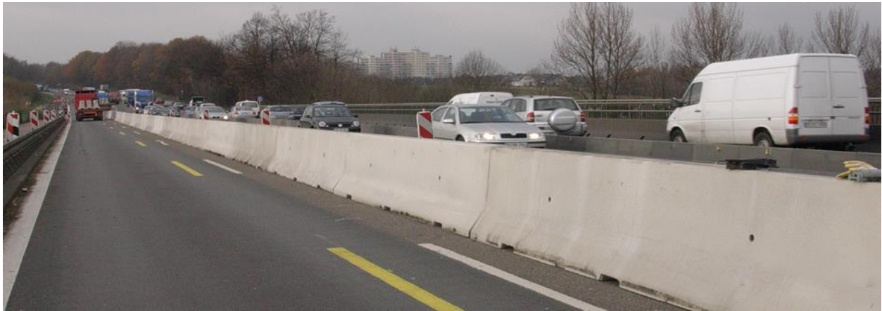
FIGURE 5 Temporary contraflow protection at level H4b/W6
