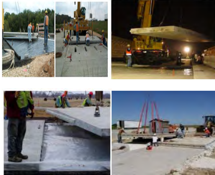
Figure 5. Precast slab projects in Texas, California, Missouri, and Iowa sponsored by the Federal Highway Administration (1).
