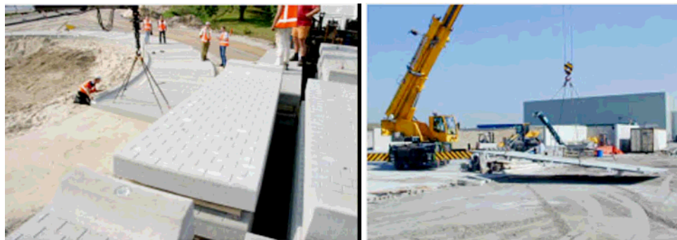
Figure 3. Precast concrete elements in a roundabout and panel lifting test in the Netherlands (12).
