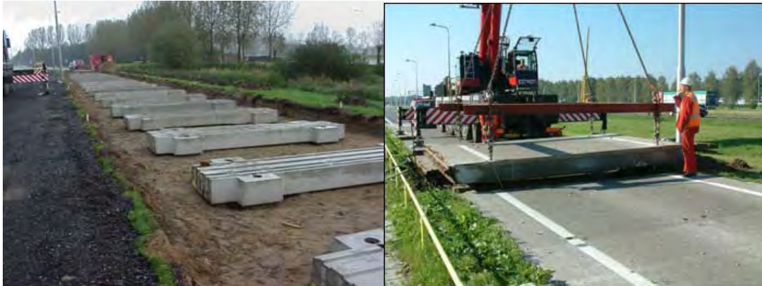
Figure 1. The ModieSlab test section along motorway A50.
