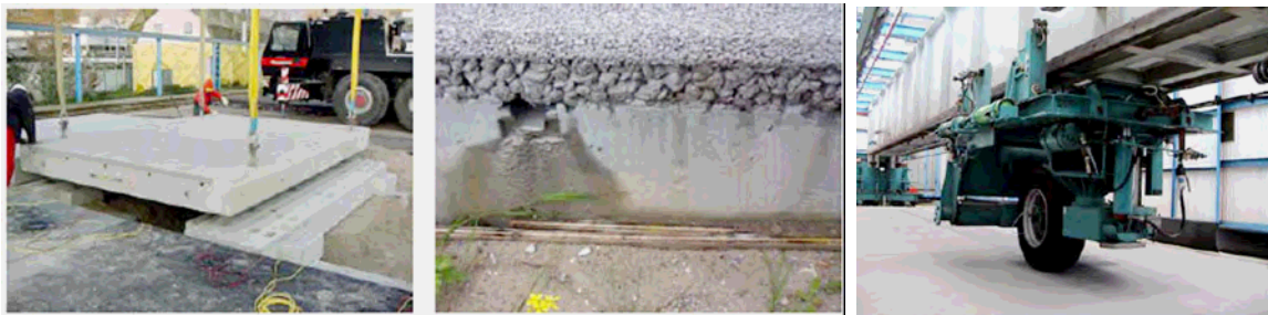
Figure 2. Construction of the ModieSlab test section for accelerated pavement testing and the LinTrack facility (9).
