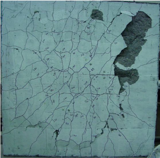
Fig. 5 Crack pattern of test slab HS4 (radial crack pattern)
