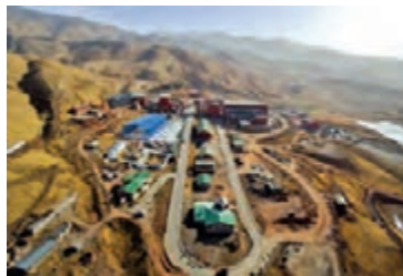
Gold processing plant
