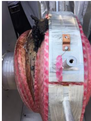
Figure 3. Internal ablation winding of A-phase PT.
