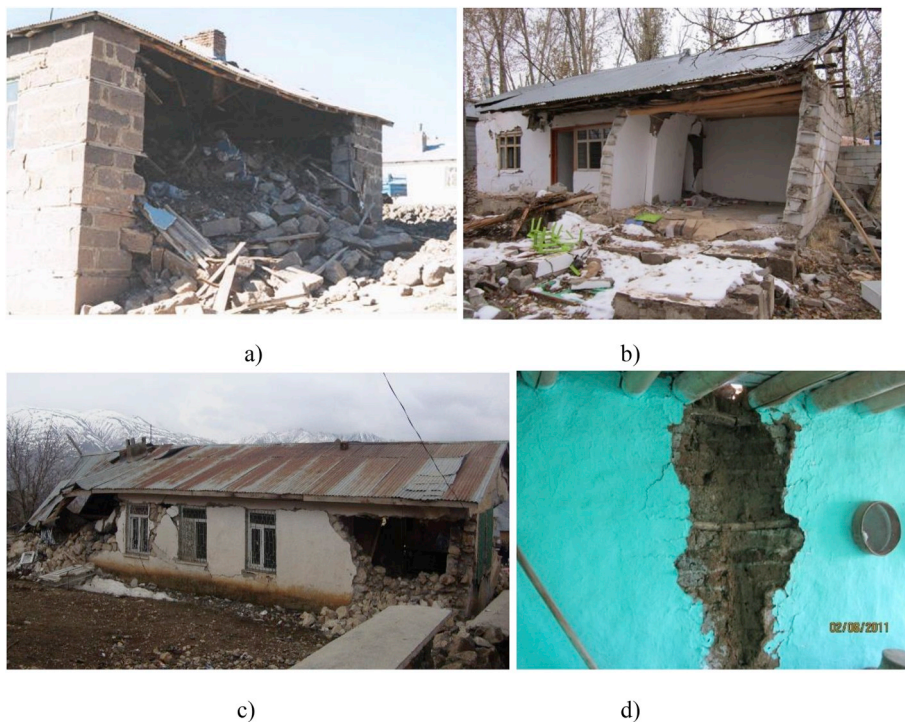
Fig. 15. Out-of-plane collapse of bearing walls in structures: (a) Bingöl (Photos by A.Karaşin, M.E. Öncü); (b) Van (Photos by B. Yön, M.E.Öncü); (c) Kovancılar (Photos by B. Yön, M.E.Öncü, A.Karaşin); (d) Maden (Photos by B. Yön).
