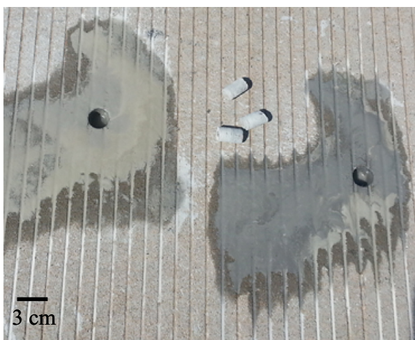
Fig. 3. Example of cores were taken from bridge deck.
