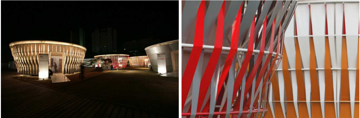
Fig. 6. (a) PVC/PES and open mesh membrane cladding for pavilions; (b) Mobile Spaces: Interwoven PVC/PES membrane strips.
