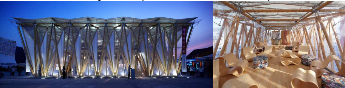
Fig. 7. (a) Bamboo Pavilion for Expo in Shanghai; (b) Transparent ETFE façade, Bamboo Pavilion for Expo in Shanghai.
