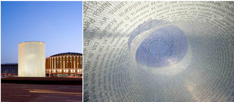
Fig. 9. (a) M11 Memorial in Madrid, solid glass blocks with inner ETFE foil; (b) M11 Memorial in Madrid, printed ETFE pneumatic structure.
