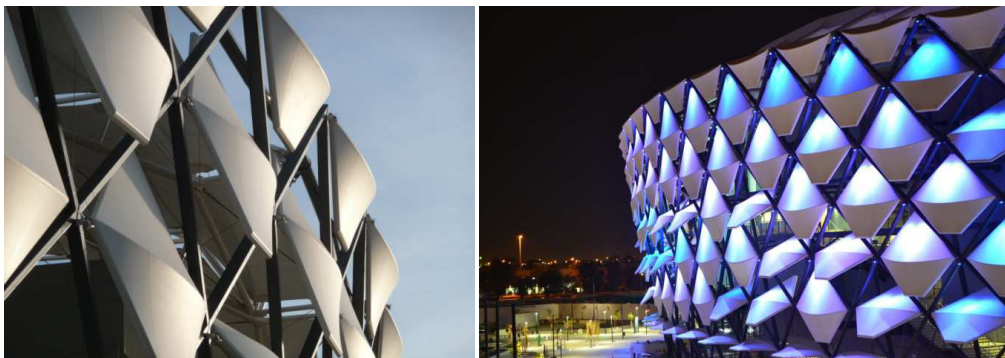
Fig. 1. (a) Glass/PTFE panel for external shading; (b) Illuminated membrane panels.
