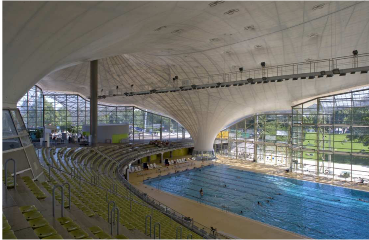
Fig. 8. Olympic Aquatic Center, Munich.
