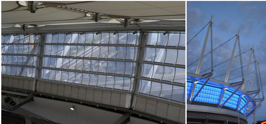
Fig. 4. (a) ETFE façade, BC Place; (b) Illuminated ETFE façade, BC Place.
