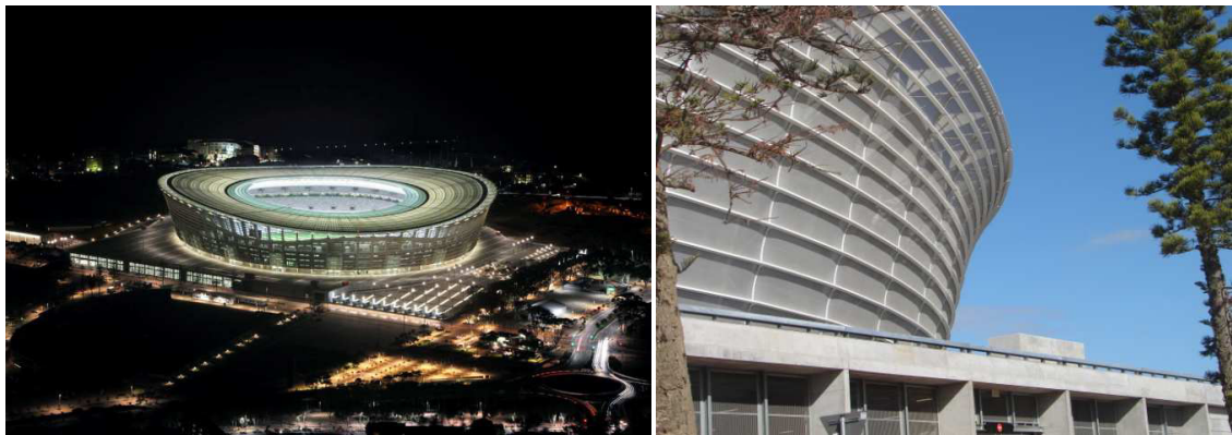
Fig. 5. (a) Greenpoint Stadium, Capetown/South Africa; (b) open mesh membrane facade.
