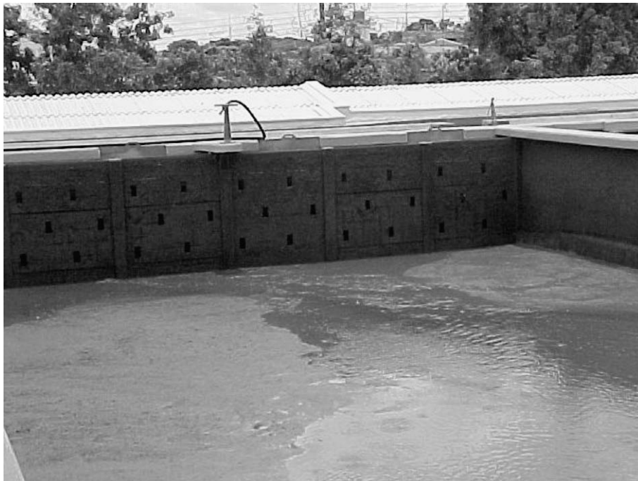
Fig. 4. State of the sludge at the moment of collection.
