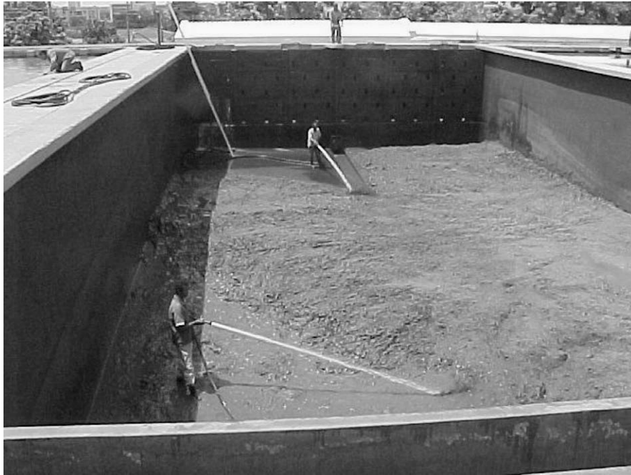
Fig. 3. Cleaning staff inside a decantation tank.
