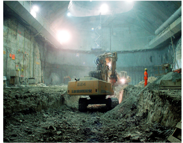
Fig. 3. Excavation of the cavern UX15 at Point 1 (ATLAS).
