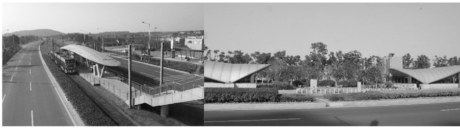
Fig. 16. Access to the SND tram: examples of an overpass bridge (left) and underpass tunnel (right). Source: Author (left) and Huahui Ai (right)
