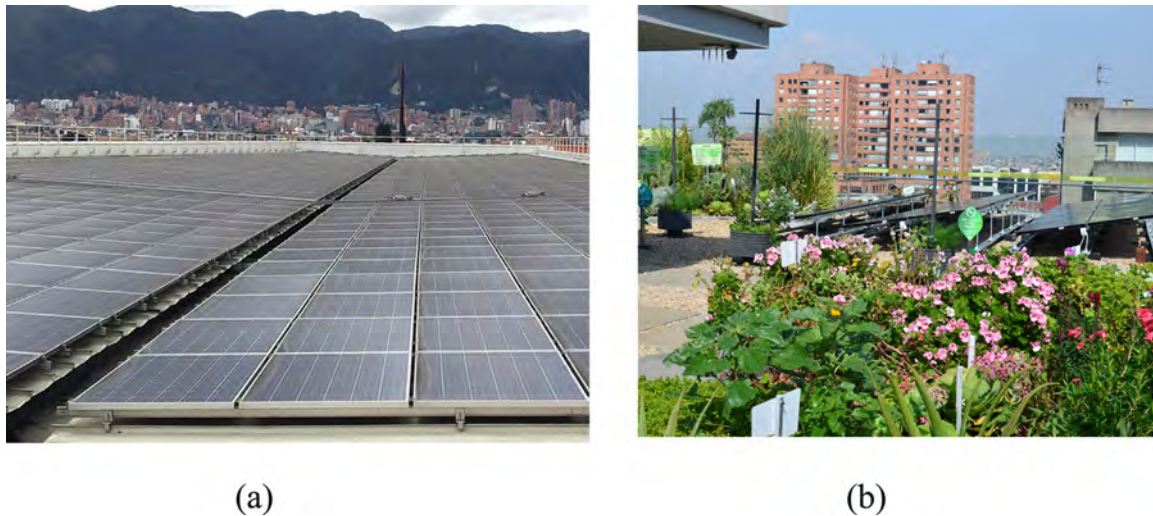
Fig. 4. Solar PV installation in Bogotá. (a) Alkosto (b) EAN University. Own pictures.
