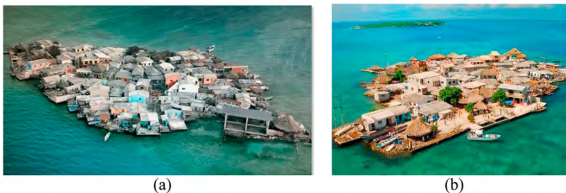
Fig. 8. Solar PV installation. Santa Cruz del Islote, Bolivar Department.
