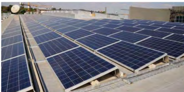
Fig. 5. Solar panels installation – EXITO Store.
