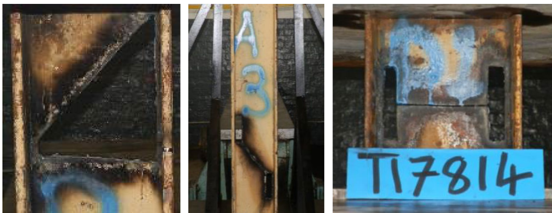
Fig. 3 Cuts made in columns using an oxyacetylene torch, showing damage to steel in the vicinity of cuts (Reproduced with permission from van Helsdingen 2012)
