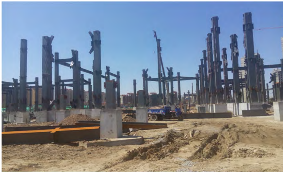
Fig. 2. The construction site of Tianjin Wanhui Square Project.
