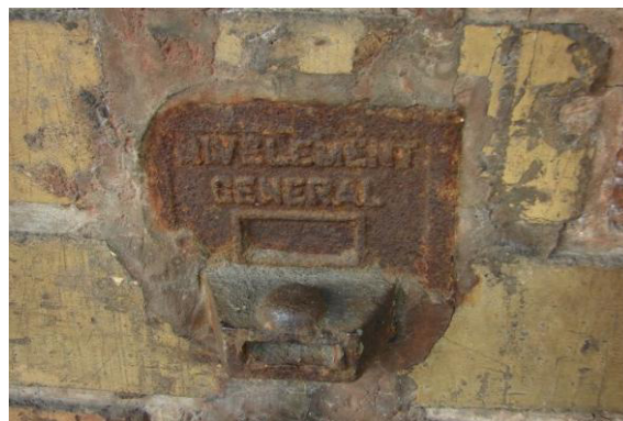
Fig. 2 Romania, landmark for the reference level \pm 0.00 , Black Sea [Credit: 3xforum topographer]
