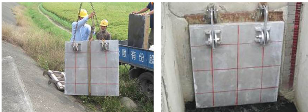
Fig. 12. Installation of Tanduliao sluice gate.
