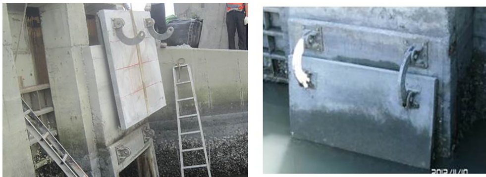
Fig. 11. Installation of Houanliao sluice gate.
