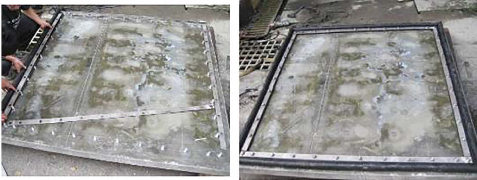
Fig. 6. FRC sluice gates installation water seal.
