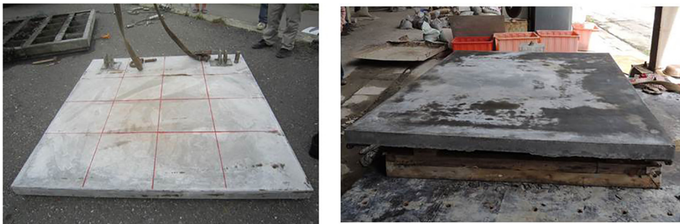
Fig. 7. Surface of the demolded FRC sluice gates.
