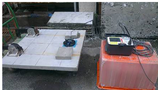
Fig. 19. Assessing corrosion in FRC sluice gates.
