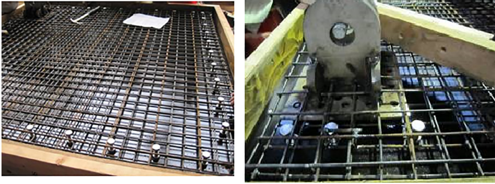
Fig. 4. Locations of lifting lugs in relation to the wire mesh.
