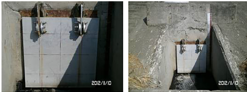
Fig. 14. The appearance of the Tanduliao sluice gate (after 12 months of field testing).
