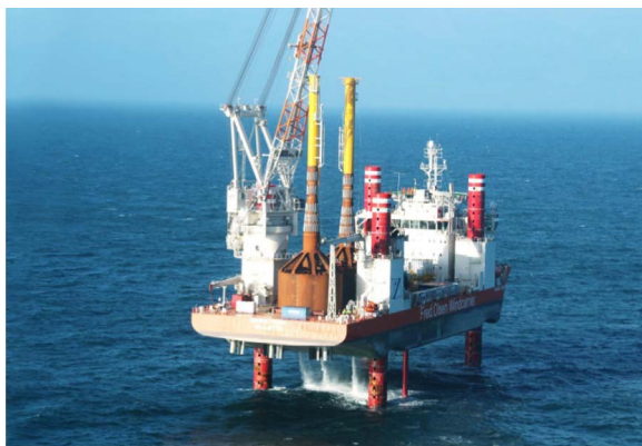
Fig. 2. Prototype Bucket foundation prior to installation.
