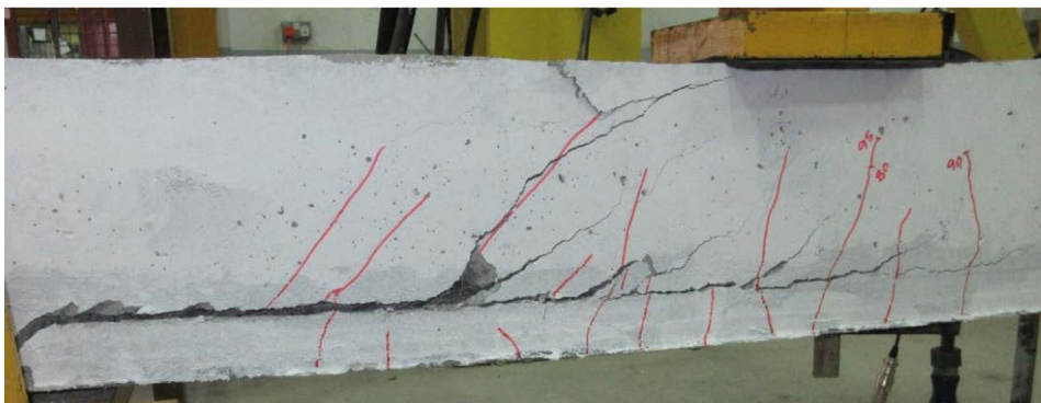
(c) S4H beam failed by end concrete cover separation
