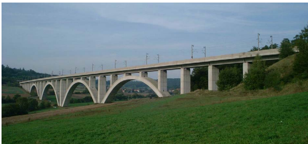
Fig. 9. Wälsebach Viaduct (Photo: Klaus with K).
