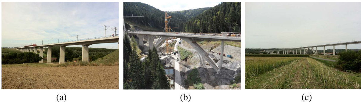
Fig. 14. Integral and semi-integral bridges on German HSR lines (a) Scherkonde Viaduct, (b) Gruben Viaduct and (c) Unstrut Viaduct.
