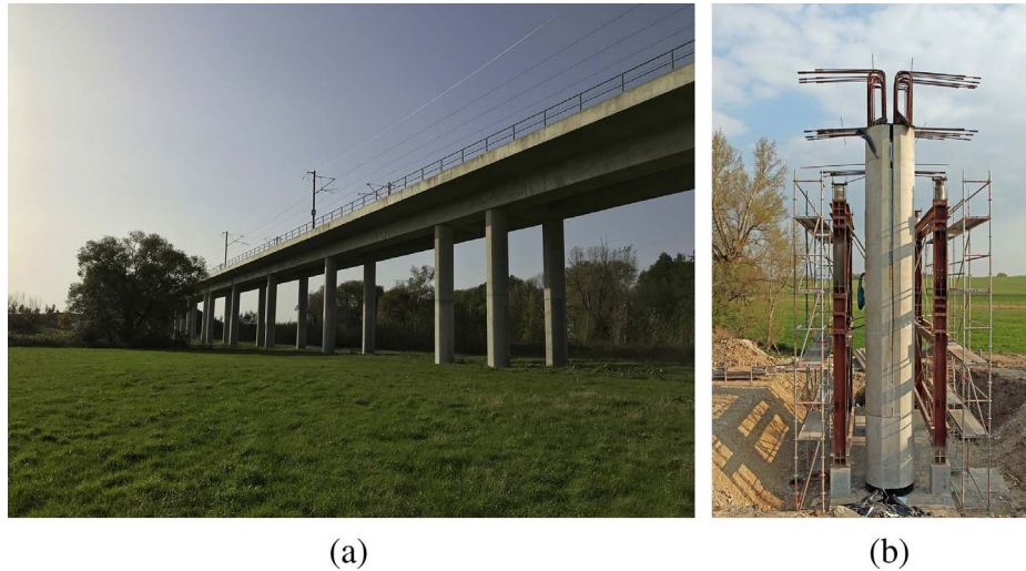
Fig. 15. Stöbnitz Viaduct (left); Sliced pier between frames (Right photo: störfix).
