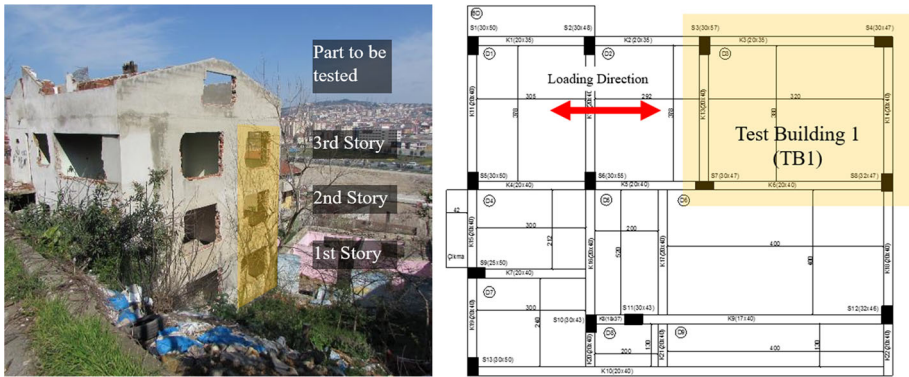
Fig. 1 General view of the test site and plan of the existing building
