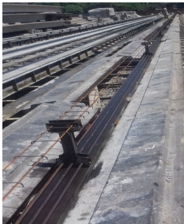
Fig. 3 Pretensioning by longline method
