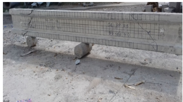
Fig. 19 Crack patterns of P6 beam
