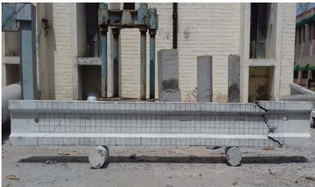
Fig. 16 Crack patterns of P3 beam
