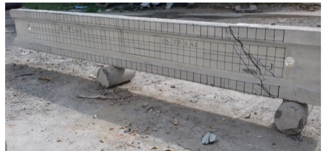
Fig. 18 Crack patterns of beam P5
