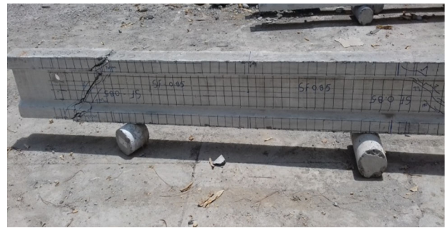
Fig. 17 Crack patterns of P4 beam
