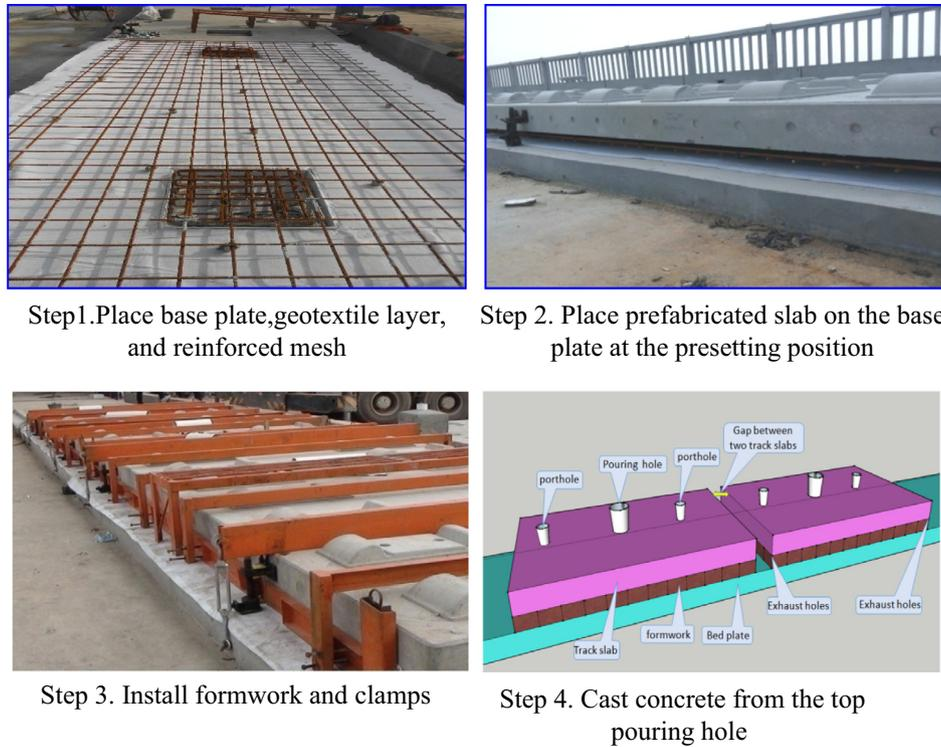
Fig. 2. The main construction steps of CRTS III slab ballastless track.
