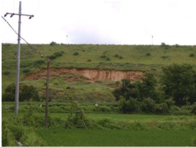
Fig. 4. AG dam incident: downstream slope failure (2003).
