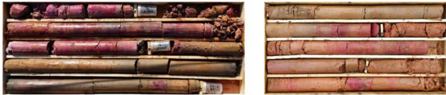
Fig. 15. Chemical indicator reaction for HD dam checkhole core samples after remedial grouting.
