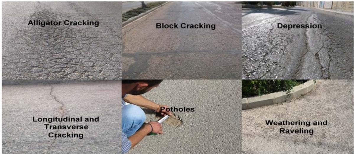
Fig. 4. Examples of pavement distress types from the site of study.
