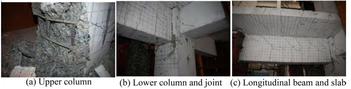
Fig. 7. Failure modes of specimen C.
