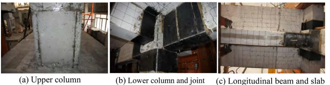
Fig. 10. Failure modes of specimen SCBW.
