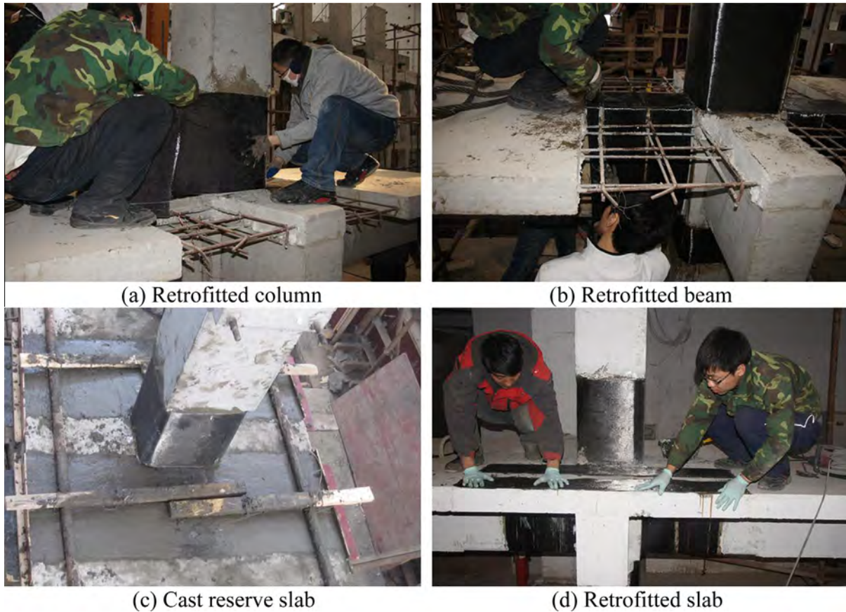
Fig. 3. Pictures showing retrofitted process of specimen SCBW.
