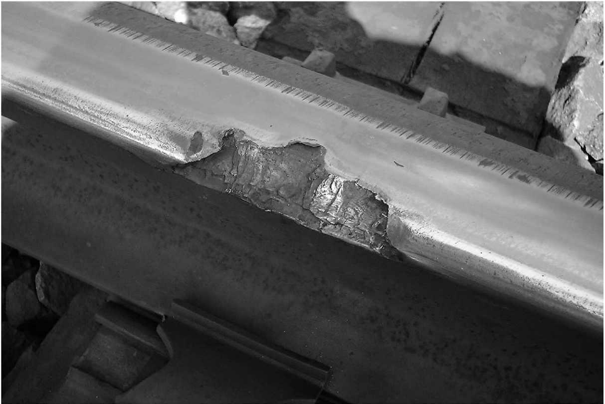
Fig. 1. Example of severe localised spalling on Malmbanan.
